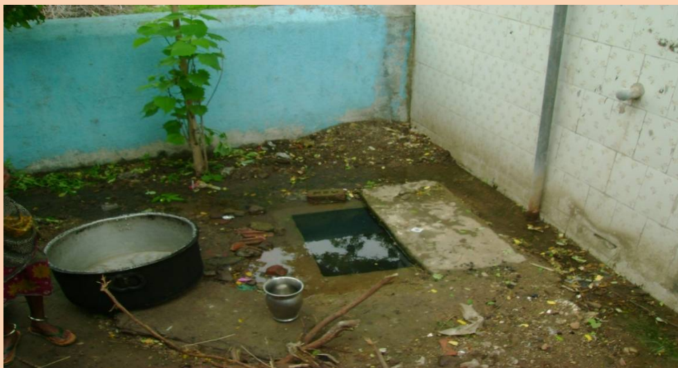
(lack of maintenance of the premises for preparing mid day meal – the place is unhygienic)
