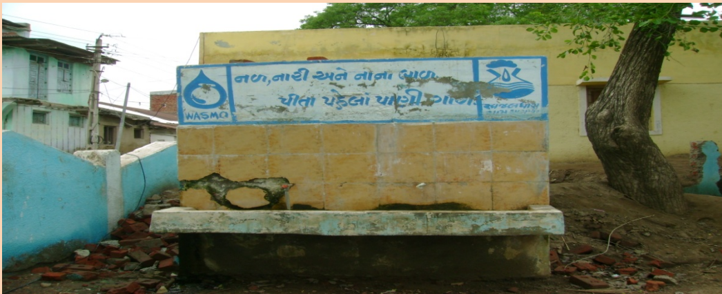
(The surroundings of the drinking water facility are unhygienic)
